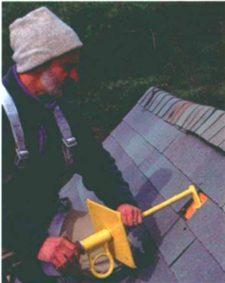
A good anchor attaches snugly to the rafter. The author first removed a layer of shingles and drilled a hole in the roof to attach this roof anchor to a rafter. The L-shaped end of the anchor is fed through the hole and secured around the bottom of a rafter. A large wing nut on the threaded shaft is tightened down over a steel plate to fasten the anchor firmly to the roof.
